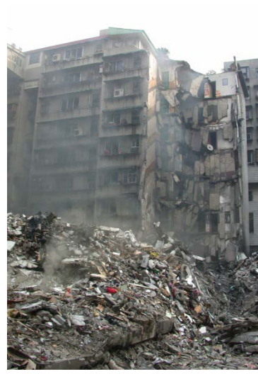
(b) The southeast side of the building
