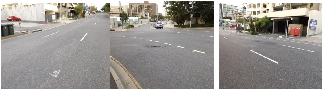
Figure 5.40: Deterioration of surface condition and pavement repair of flood affected parts of Cordelia Street, South Brisbane (pictures taken in 2015)
