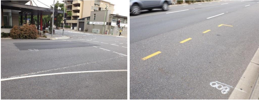
Figure 5.41: Pavement repairs due to surface condition deterioration of flood affected parts of Cordelia Street, South Brisbane
