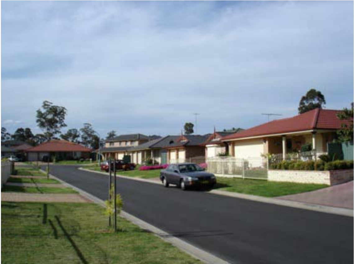
Figure 7 - The street scene in a cul-de-sac off Meacher Street, Mount Druitt NSW. Note the dominance of the garage doors.
