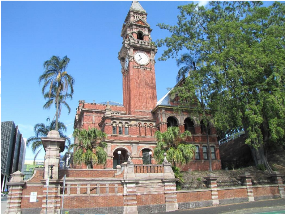
Figure 2 South Brisbane Municipal Chambers, 2017 (Source: Author)
