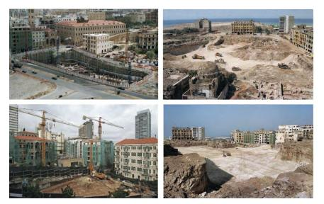
**Figure 70:** Selected photographs showing excavated holes in Beirut in preparation for future buildings. From Solidere, The Chronicle (Lebanon, 2012).
