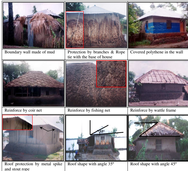
Figure 7 Indigenous knowledge practiced by local communities for the protection from disaster (Ahsan and Azam, 2007).
