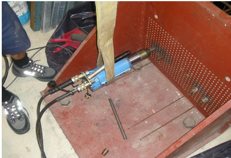
Figure 2 Applying of prestressing force using hydraulic jack in progress
