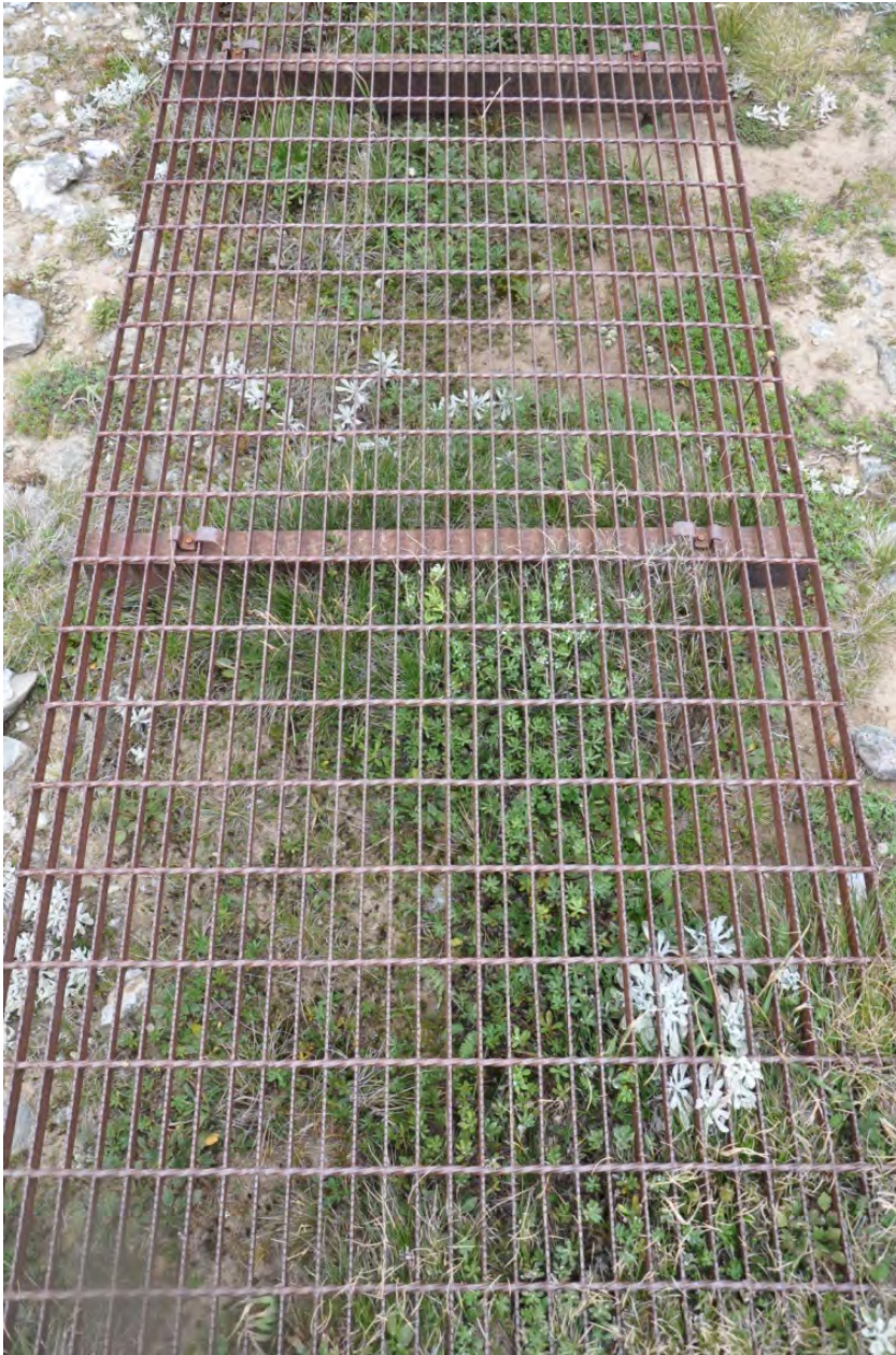
Figure 5: Example of a steel metal walkway constructed in 1998 as a trial to observe the effects of elevating recreational trampling. The walkway is constructed from ungalvanised 'cut corrugated grip' steel mesh and seems to facilitate the establishment of many Feldmark plants. (Photo: Mark Ballantyne).
