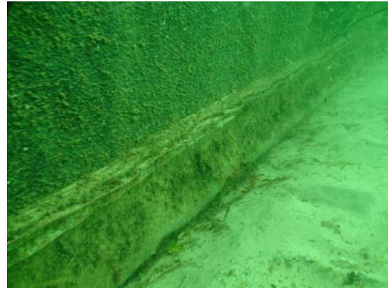
Figure 17: Seabed based algae curtain resting on seafloor
