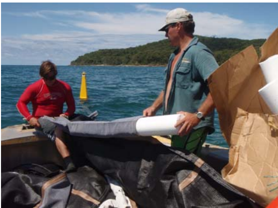
Figure 16: Final assembly and deployment of algae curtain
