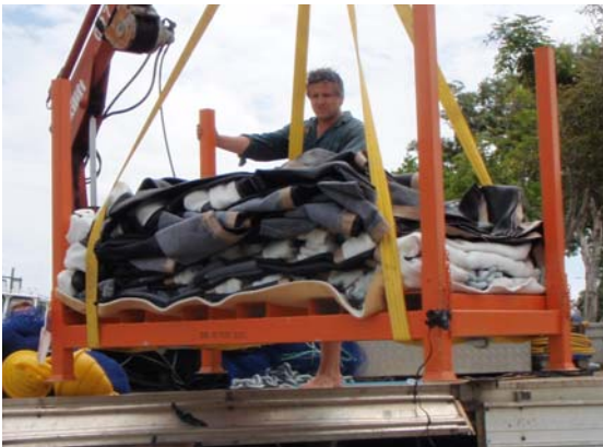
Figure 15: Seabed based algae curtain prior to installation
