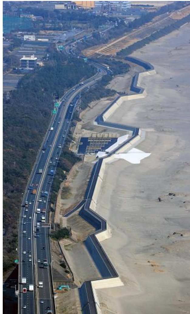
Fig. 1: Breakwater along the coastline in Hamamatsu, Shizuoka Prefecture, Japan (Photo by Hikaru Uchida/The Asahi Shimbun via Getty Images)
