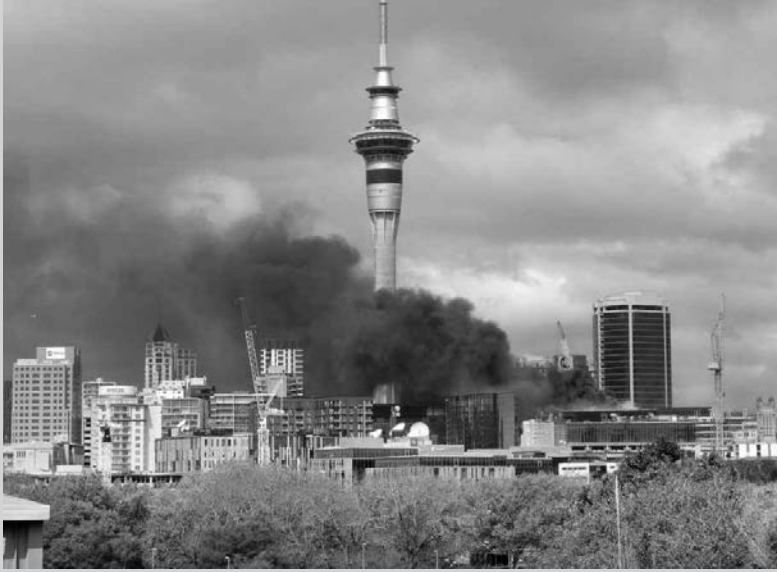
Figure 5.1: SkyCity Convention Center Roof Fire and Sky Tower.
