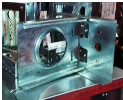
45 Fig 1: Cold-formed steel channel with a stiffened web hole.
