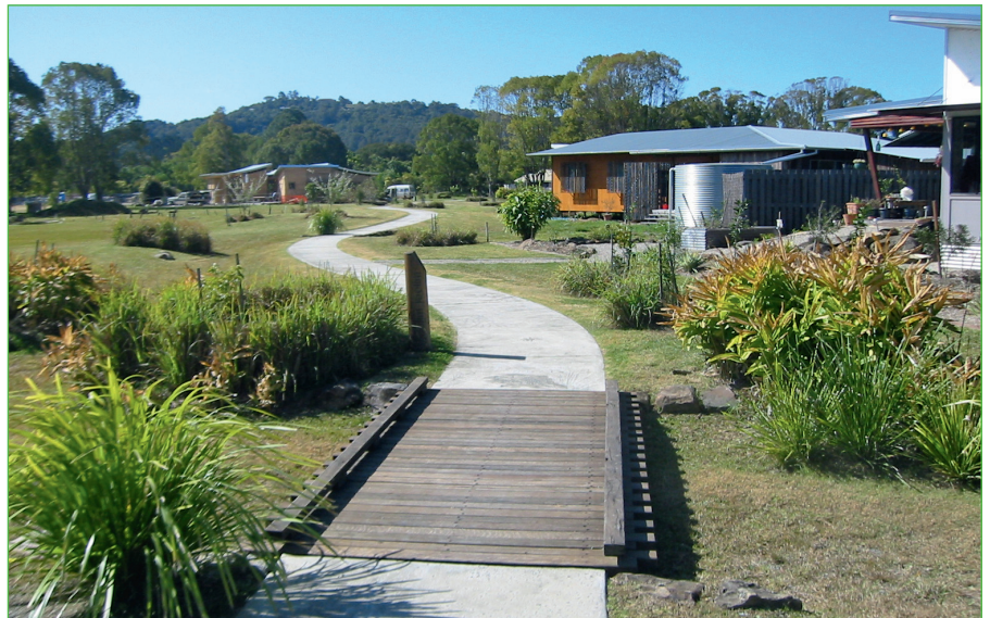
Typical pedestrian friendly layout of The Ecovillage homes showing high communal open space with quality landscaping, climate adaptive housing and rainwater tanks.
