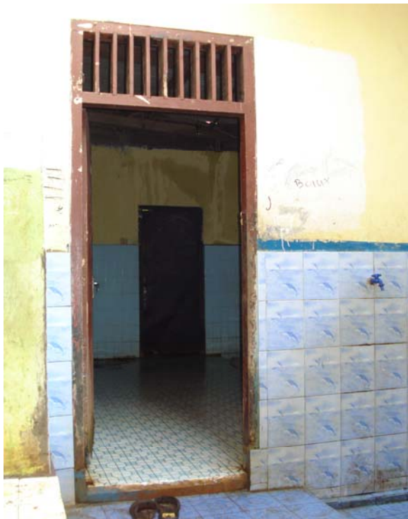
Figure 7.4. Toilet for students in School B
