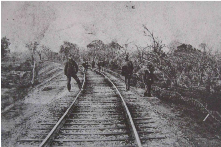
1.4 Repaired railway outside of Glenrowan, 1880. (McMenomy 1984, p. 167)
