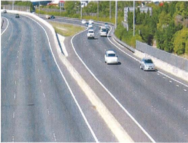
Figure 2.2 Road section exhibiting level of service B
