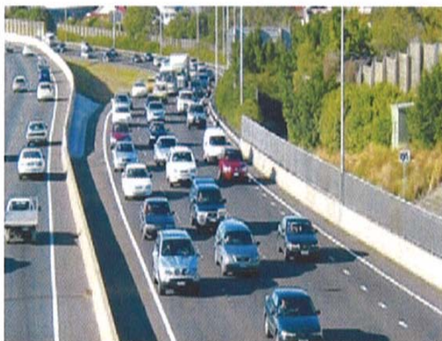
Figure 2.6 Road section exhibiting level of service F
