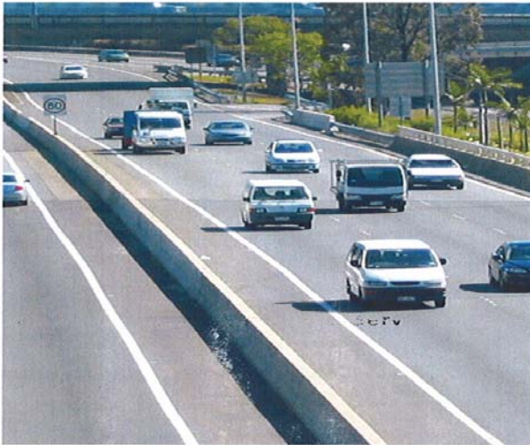
Figure 2.4 Road section exhibiting level of service D
