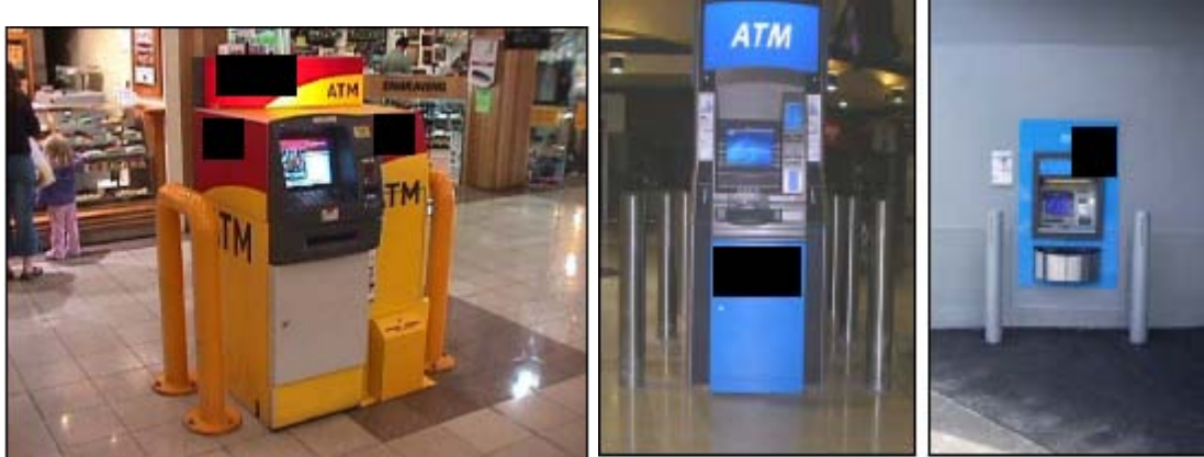
Figure 1: Examples of Internal Bollards and Barriers
