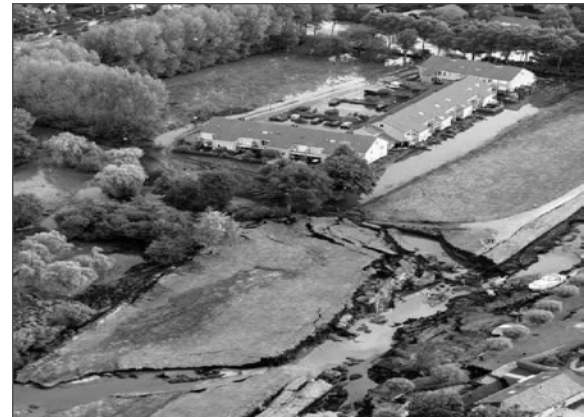
Fig. 3 Wilnis dyke the morning after [19].
