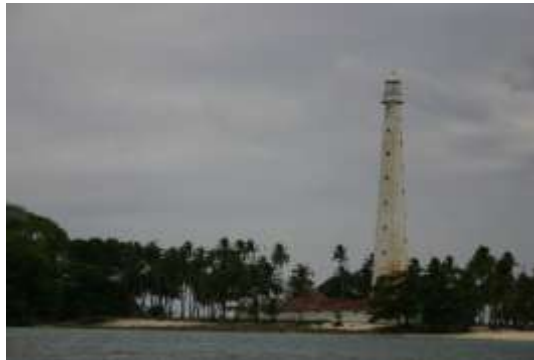
Figure 7. Lengkuas island lighthouse (source: Balar Sumsel)
